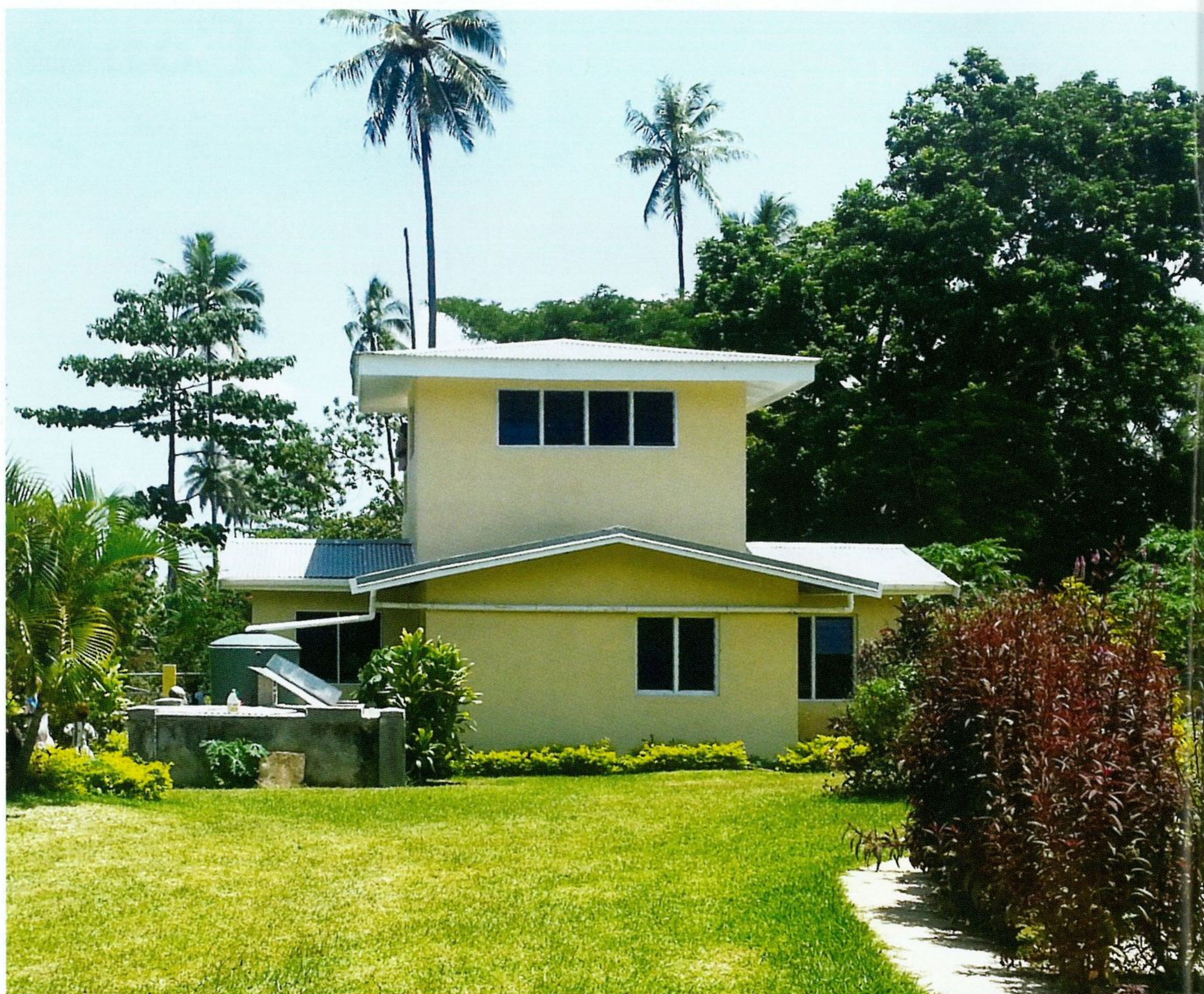
The main office building
